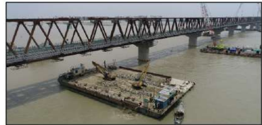
Dumping Barge at Bangabandhu Rail Bridge
